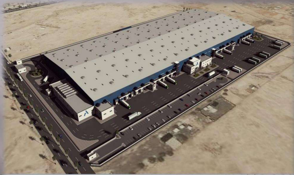
Riyadh warehouse site
